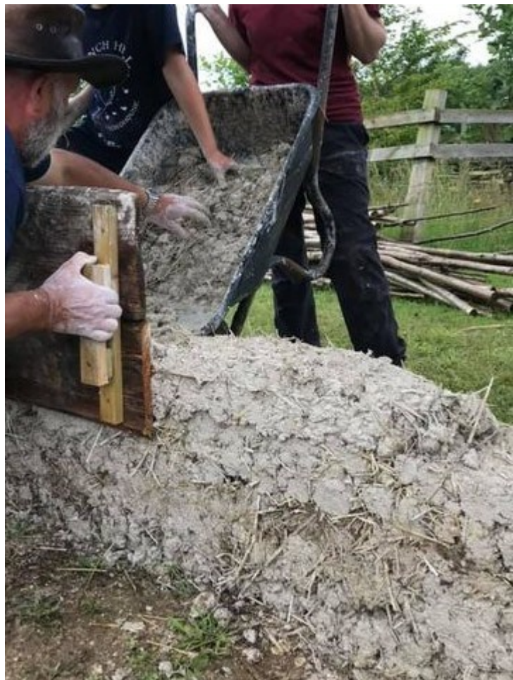
Fig. 4: Constructing chalk cob wall (Butser Ancient Farm 2021).
