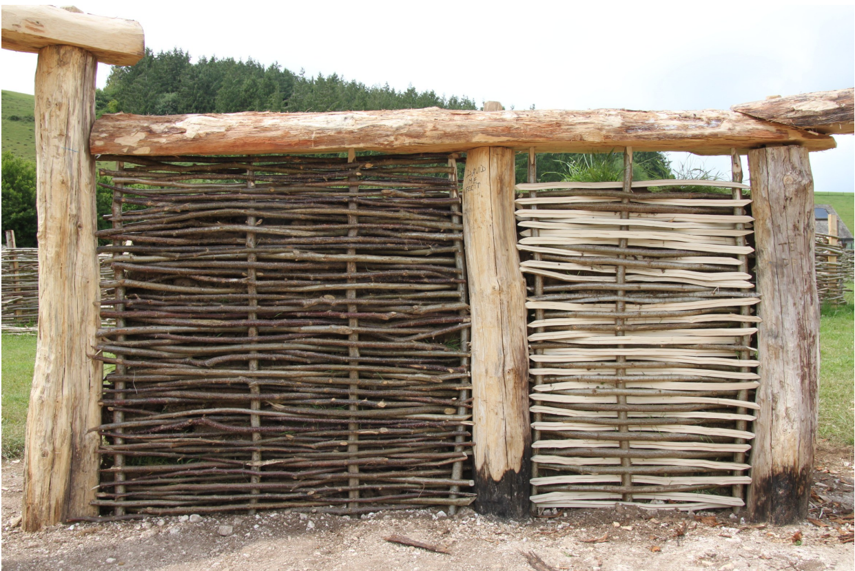
Fig. 2: Post and lintel frame with wattle panel revetting (photograph by the author).
